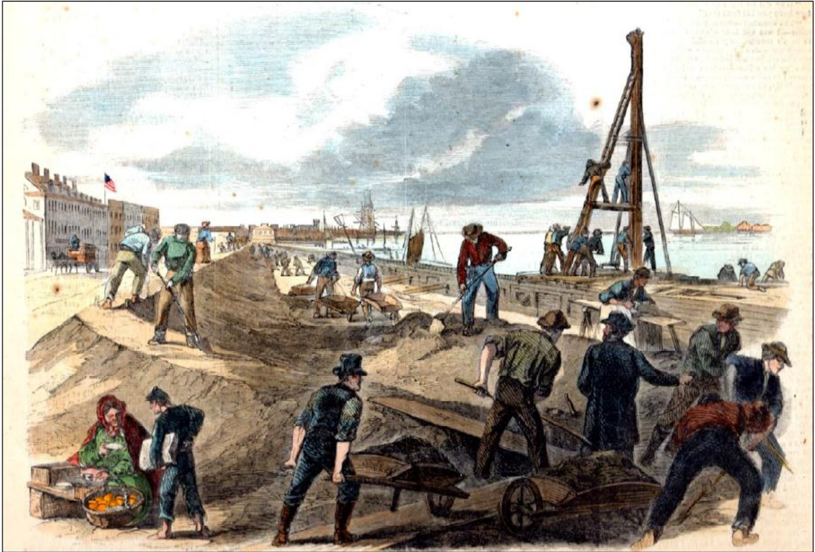
Levee construction at New Orleans in 1863, during the Civil War.
